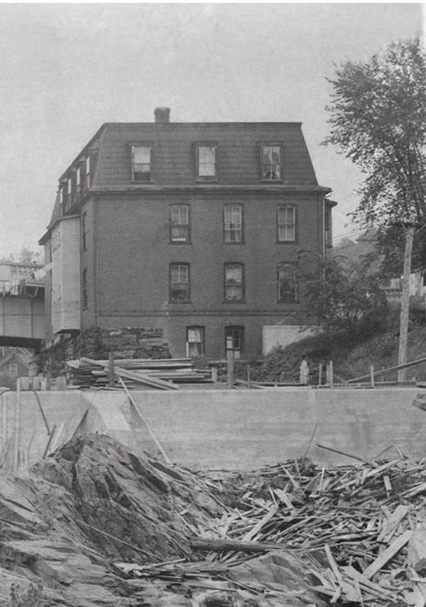
Building of the Bethel Mills Dam, summer of 1940.
