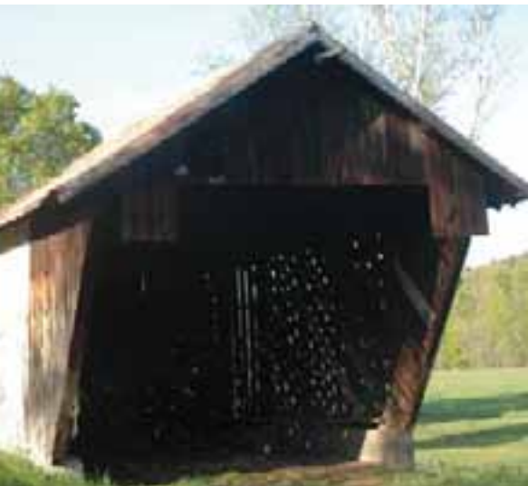
The wood drying shed.
