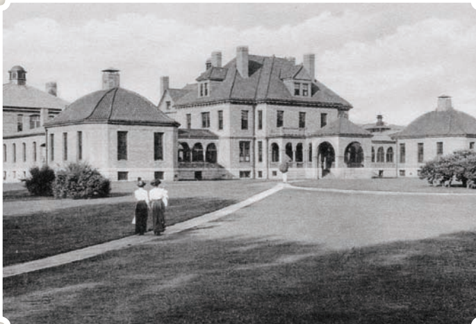
Mary Hitchcock Memorial Hospital, A&B Ward, Addition, 1913.
