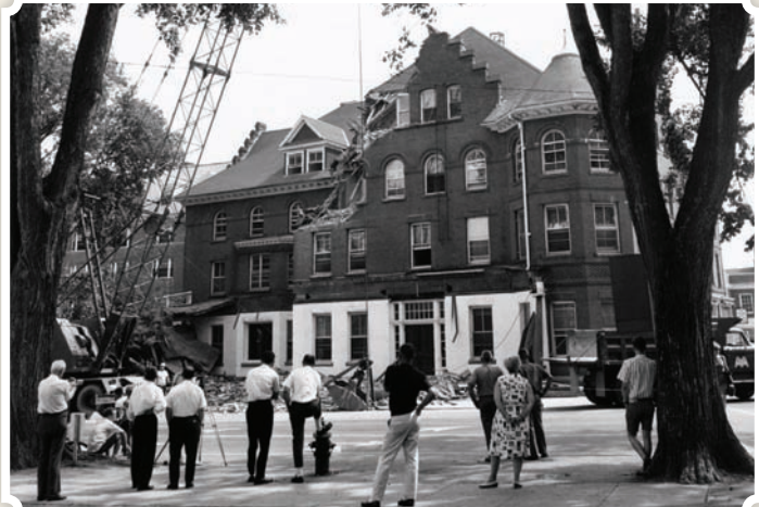
Beginning demolition of the old Hanover Inn, June 1966.
